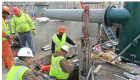
*FSI Model PP 288 Push Piers being driven around the Air Eliminator Pads through a Flush Mount Bracket.*
