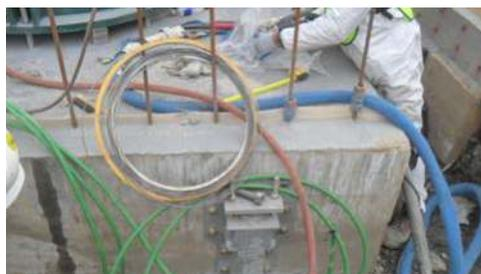
*PolyLEVEL is applied via an injection process through a series of pre-drilled holes in the Eliminator pad. These holes are methodically placed to provide fill in the proper areas.*
