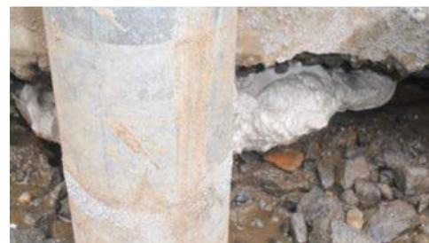
*The PolyLEVEL fill is monitored through the injection process to ensure proper application. PolyLEVEL is visibly filling gaps and crevices caused by settlement.*
