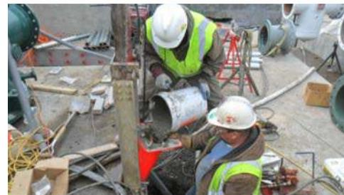
*5,000 psi mix concrete is poured into the Push Pier sleeves to add rigidity and strength.*
