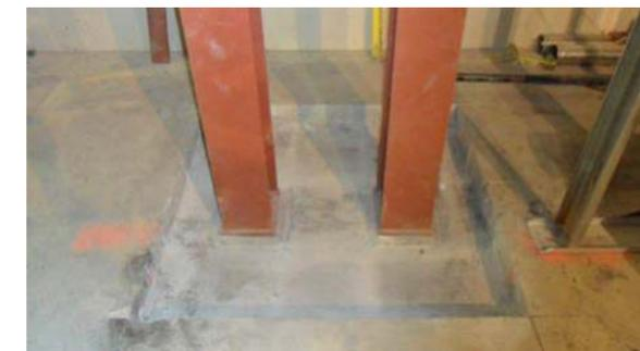
Dual beams on four helical piles providing foundation support.
