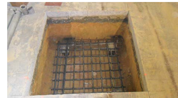
Four helicals with pile caps and rebar are awaiting concrete.
