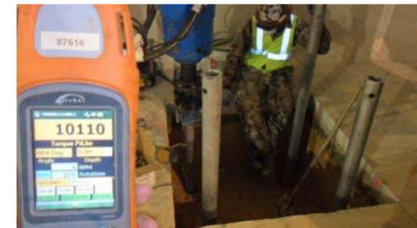
Installing four helicals to support dual beams. Pro-Dig handheld display assisting with the installation to insure lasting stability of the helical designs.
