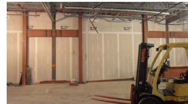
New perimeter beams on helical supported footings.
