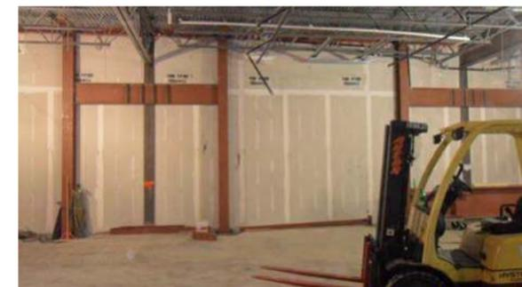
New perimeter beams on helical supported footings.
