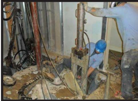
*Hydraulically Driven Pier Shafts*
